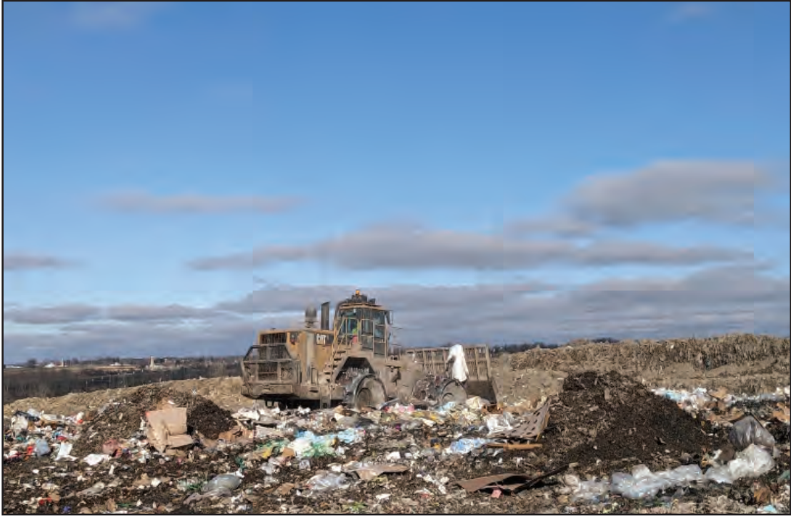
Compactor in Phase 4
