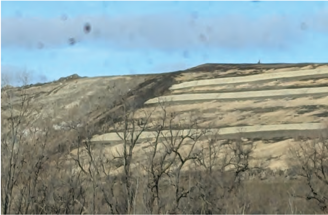
Cap project awaiting seeding and minor erosion repairs
