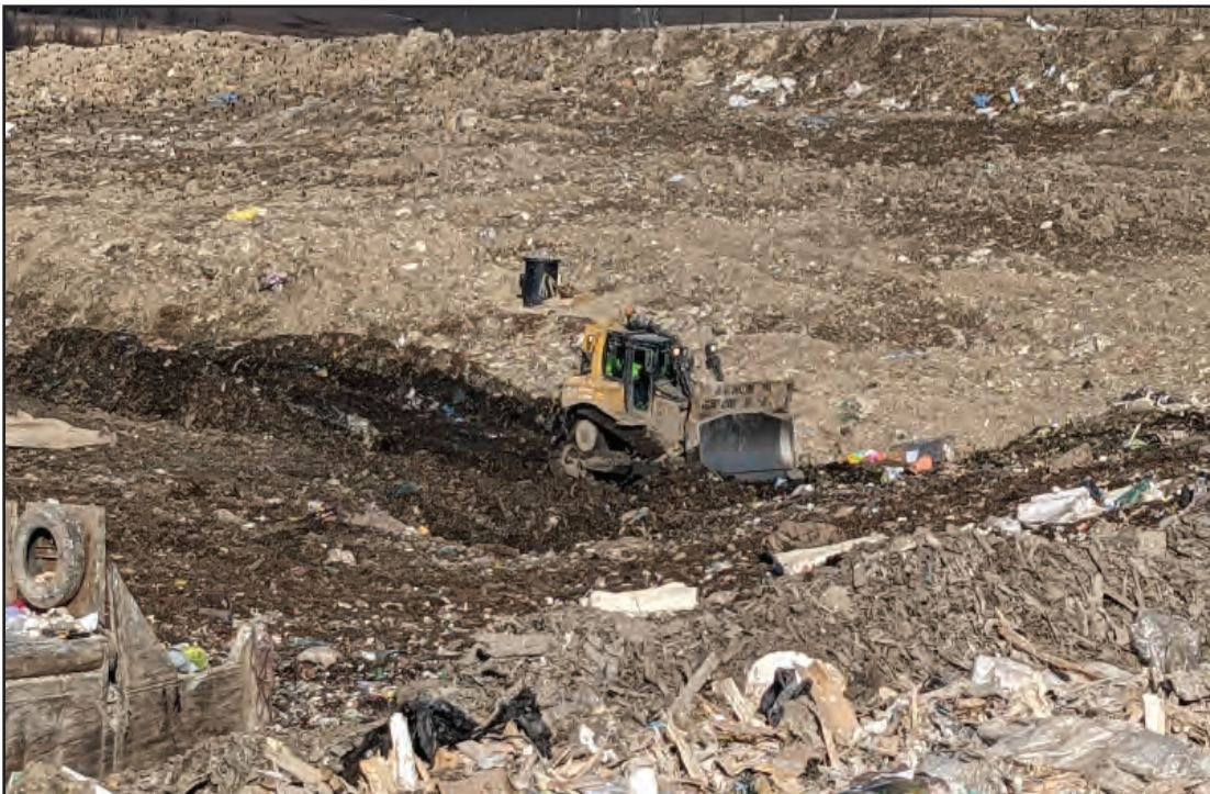
Dozer recovering cover and reshaping active area
