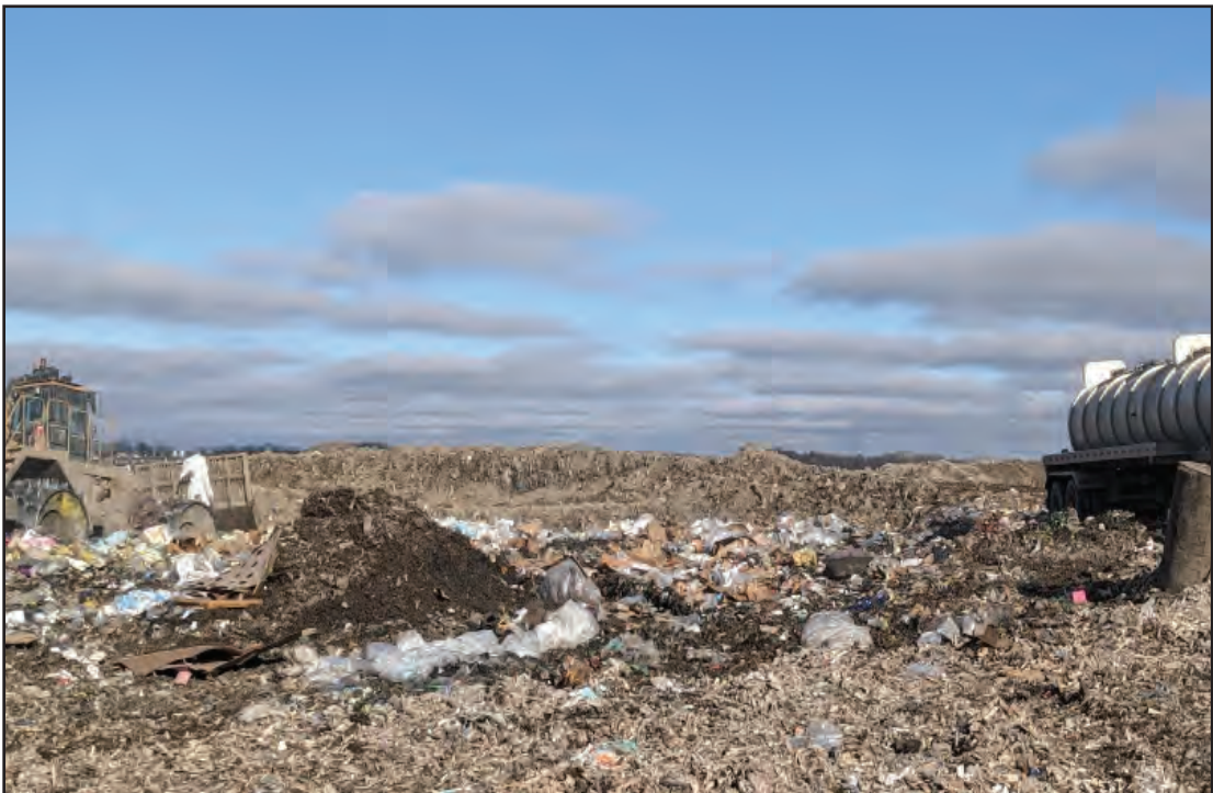
Tipping near working face
