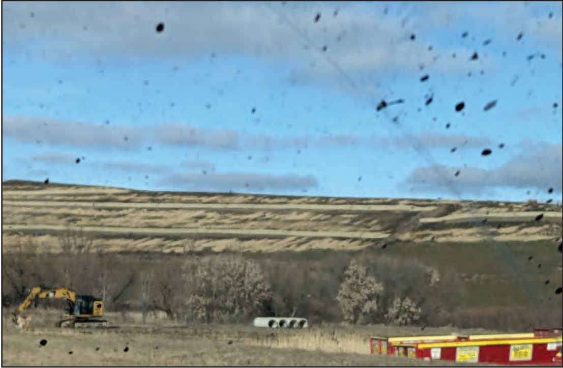
Cap project awaiting seeding and minor erosion repairs
