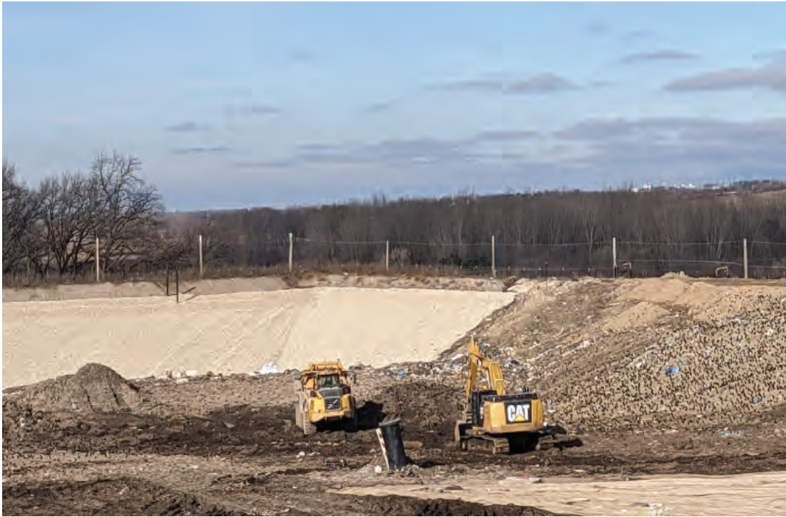
Phase 3 leveled out and stockpiles of cover placed for future waste placement
